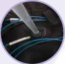
Precision volume delivery to prevent over saturation
